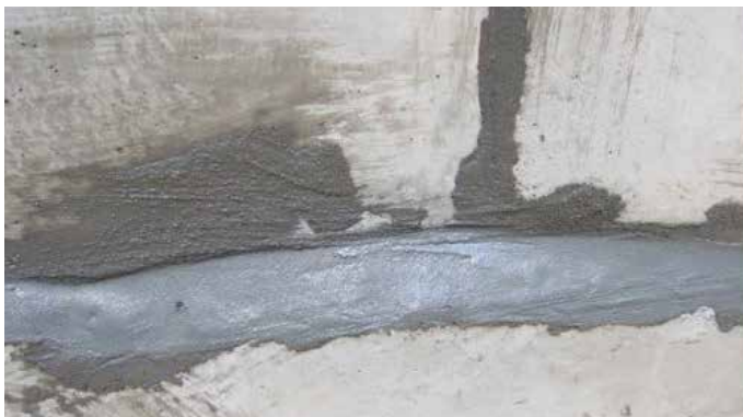
The surface is leveled using KÖSTER Repair Mortar NC. Holes and voids bigger than 5 mm have to be closed and filled with KÖSTER Repair Mortar NC.
