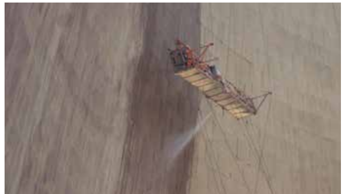
Pre-wetting the surface and application of KÖSTER NB 1 Grey in one step.
