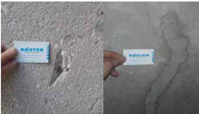
Exposed reinforcement must be cut back and covered with KÖSTER Repair Mortar NC.
